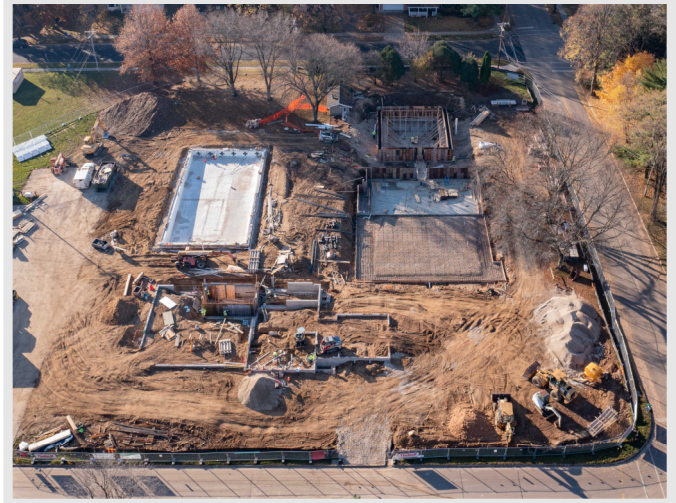
Above: Drone photo taken from Barton Rd. showing the layout of the new pool house at the bottom, existing lap pool in the top left corner, and the new dive well and competition/recreation pool in the top right corner.
